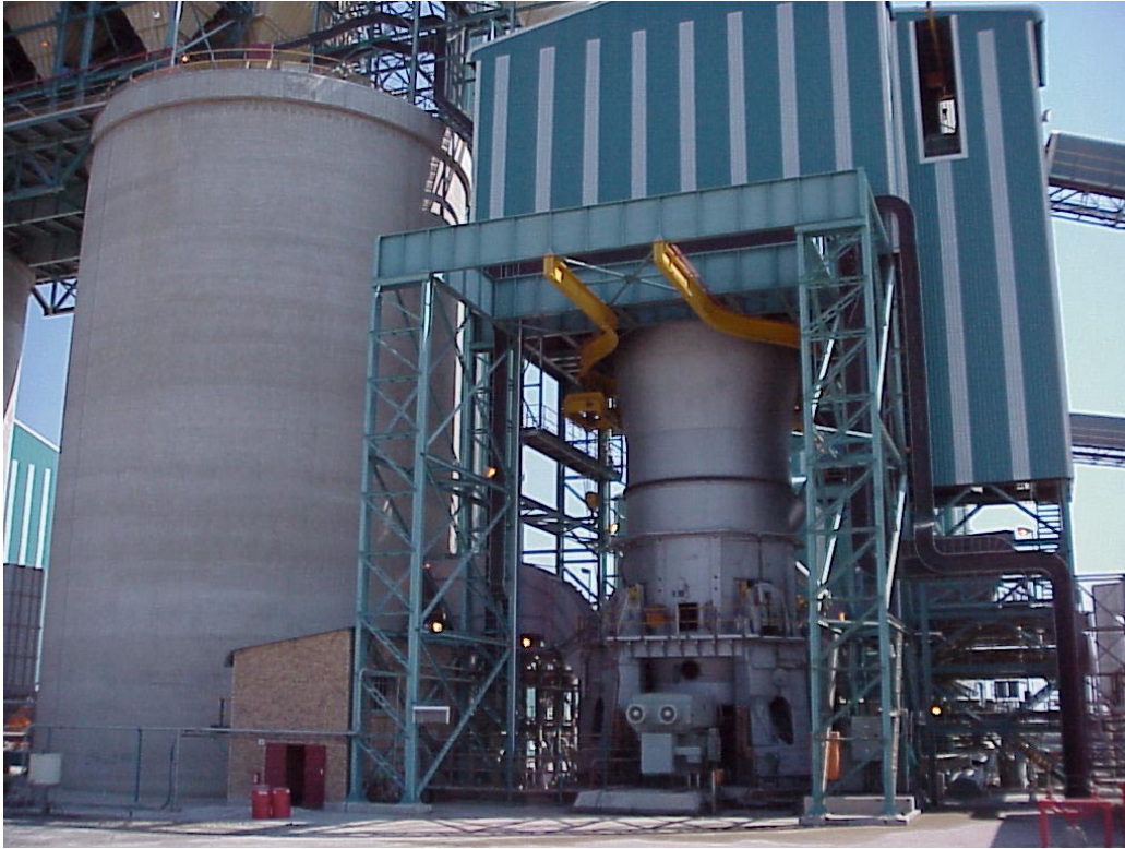
Figure 4. Latest expansion at Foskor's metallurgical facility, showing new milling technology.
